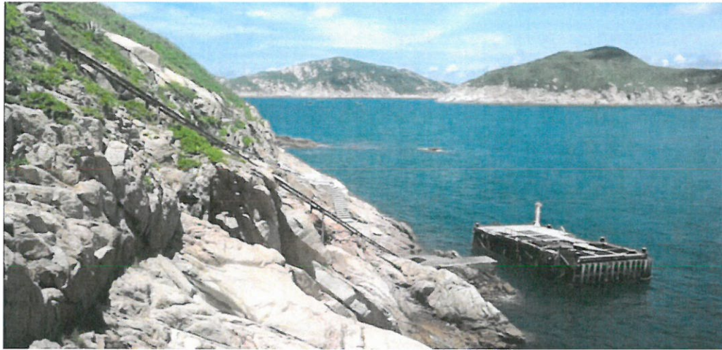
Figure 31 The Damage Pier without the Bridge (Source: Internet)
