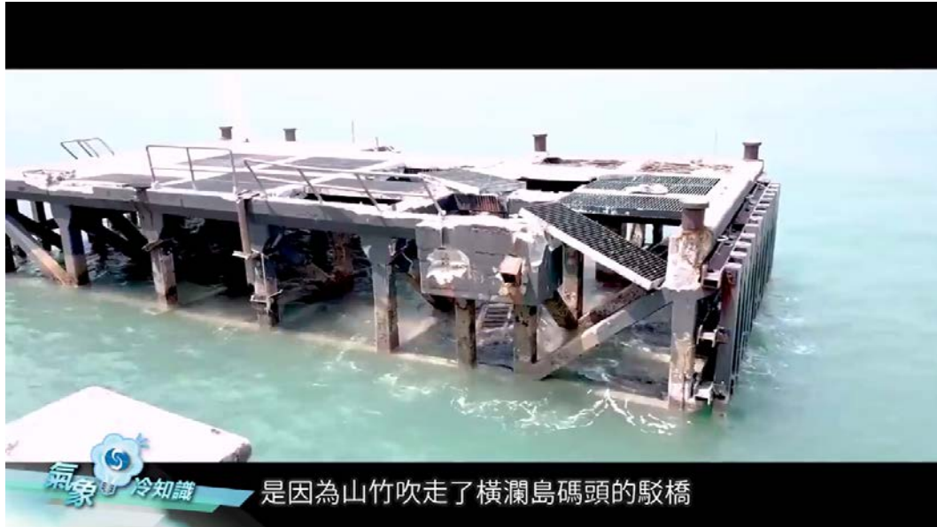
Figure 55 Typhoon Damages to the Pier and the Bridge (2018) (Source: Hong Kong Observatory)
