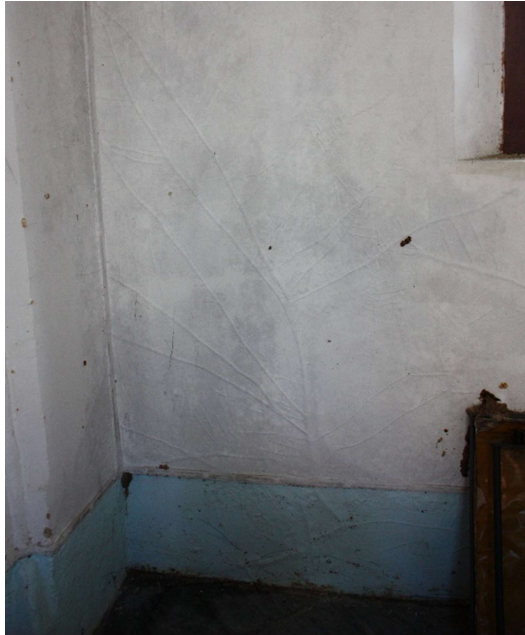
FIGURE 4-24 Tree root inside the wall
