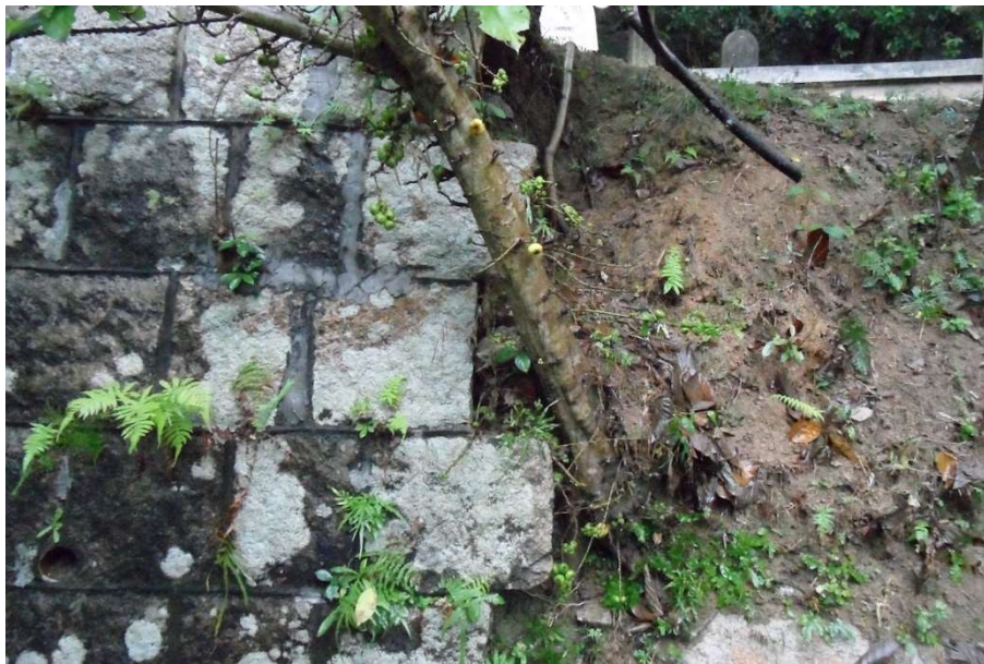
FIGURE 5-22 Cut Slope 11SW-D C 2148 Showing Wall and Soil Junction
