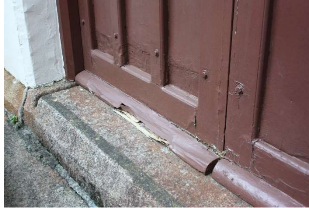
FIGURE 4-25 Timber door with signs of termite at the wooden cill
