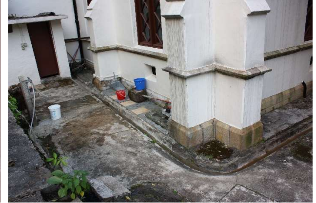
FIGURE 4-26 Use of water tap at the West side of the Chapel causes constant dampness to the historic wall
