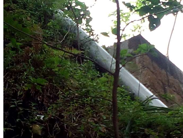
FIGURE 5-18 Downpipe from Catchpit
