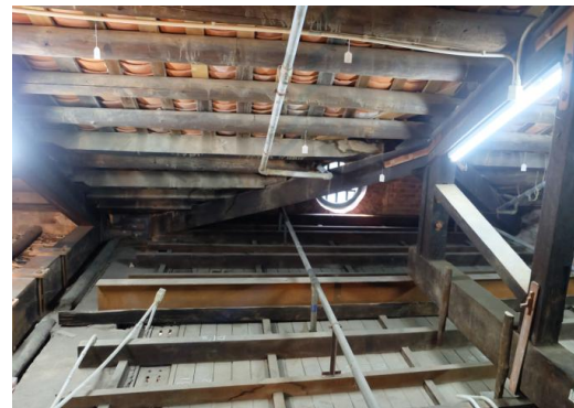
Fig.30. pan and roll tiles sitting on timber purlin and principals.
