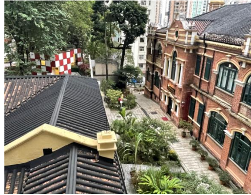
Fig. 63. Main Building is the highest in the Compound and allows sunlight to enter from the main façade side without obstruction.
