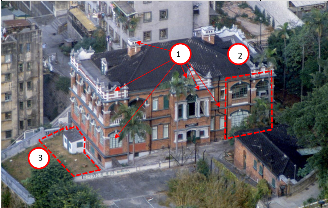
Fig. 74. Main Building in 1980s. (Source: Courtesy of Mr. Andrew Tse, for use of HKMMS in the CMP only)
