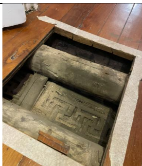
Fig. 31. timber joists under the teak floor.
