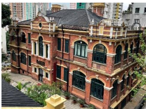
Fig. 29. Red brick external wall structural with double-pan-double-roll tiled pitched roof.
