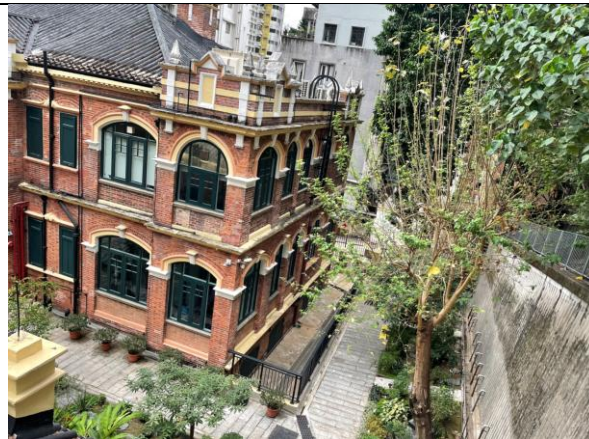
Fig. 20. Retaining wall facing south-east side of the Main Building
