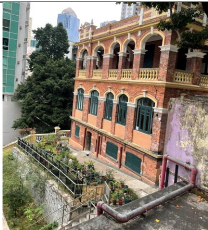
Fig. 19. Slope at the North-West side
