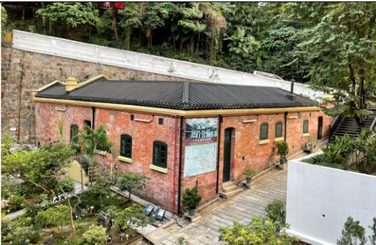
Fig. 13. Annex Block -North Corner (front view)
