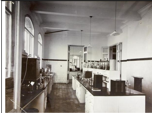
Fig. 104. Photograph of a general laboratory on the west side of the building, estimated date 1906-1910.
