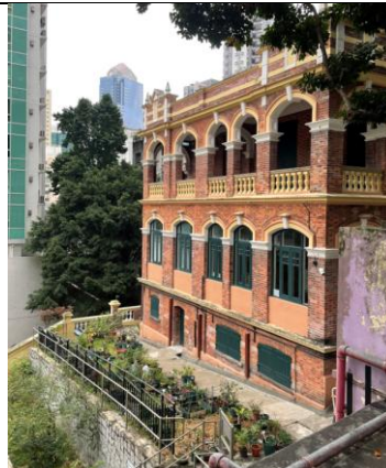
Fig. 12. Main Building -North-West side
