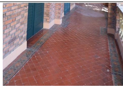
Fig. 32. Encaustic tiles flooring at the verandahs.
