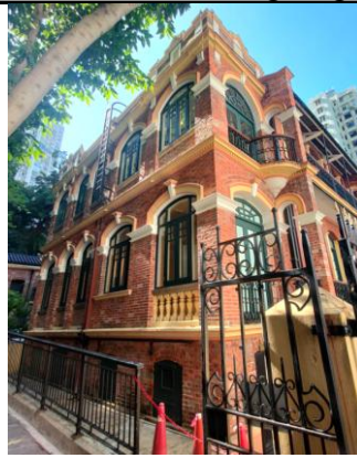
Fig. 10. Main Building -South-East Side
