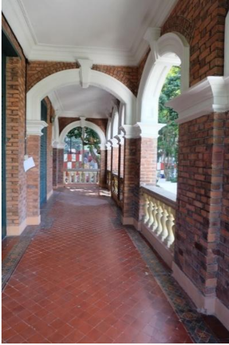
Fig. 66. Verandah and large arch opening to allow good ventilation
