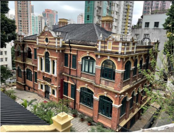
Fig. 9. Main Building -South -West Side
