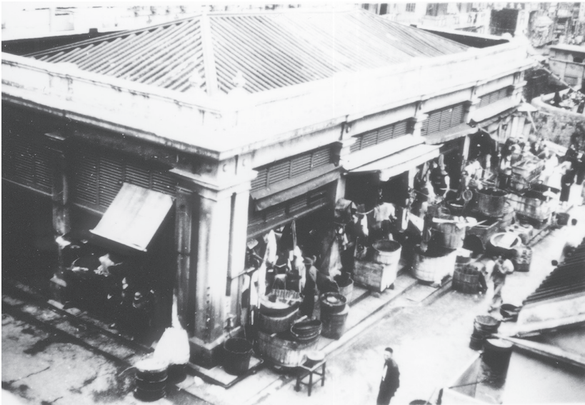
Fig. I.20. Coupled columns were used at the four corners of Shek Tong Tsui Market. (P1973.411, n.d., photograph, Hong Kong History Museum.)
