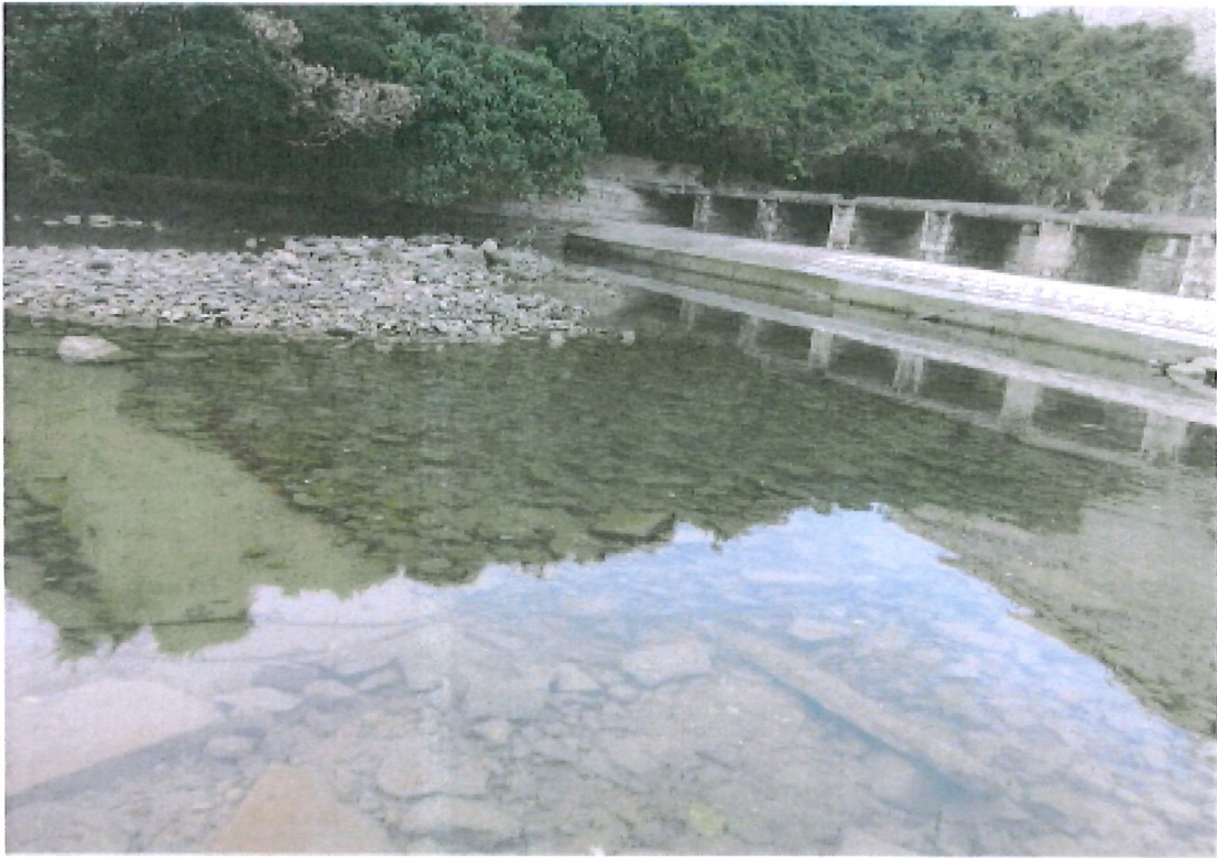
Figure 13 Cofferdam Downstream of the Dam
