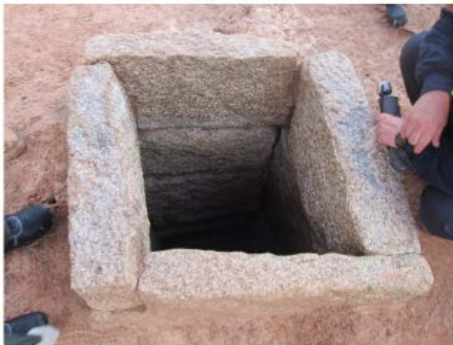
Figure 2.3 The square well is made up of granite blocks which are connected by half joints. Granite quarries should not be far away and masons are available for cutting and dressing.
