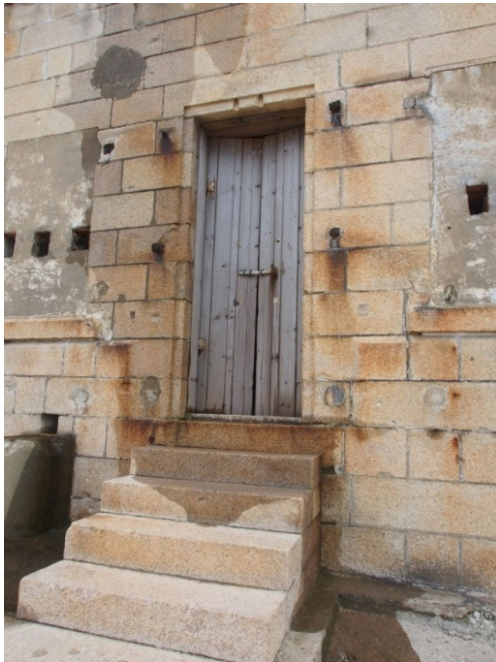
Photo 3.15 The granite facing and damages from the War
