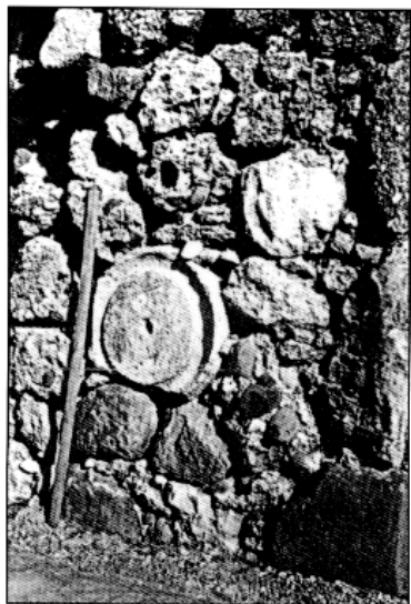
Fig. 12 Remains of grinding stone, used as a construction material for a house wall in Batanes province. It is possible that paleolithic & neolithic materials have also been recycled for house construction.
