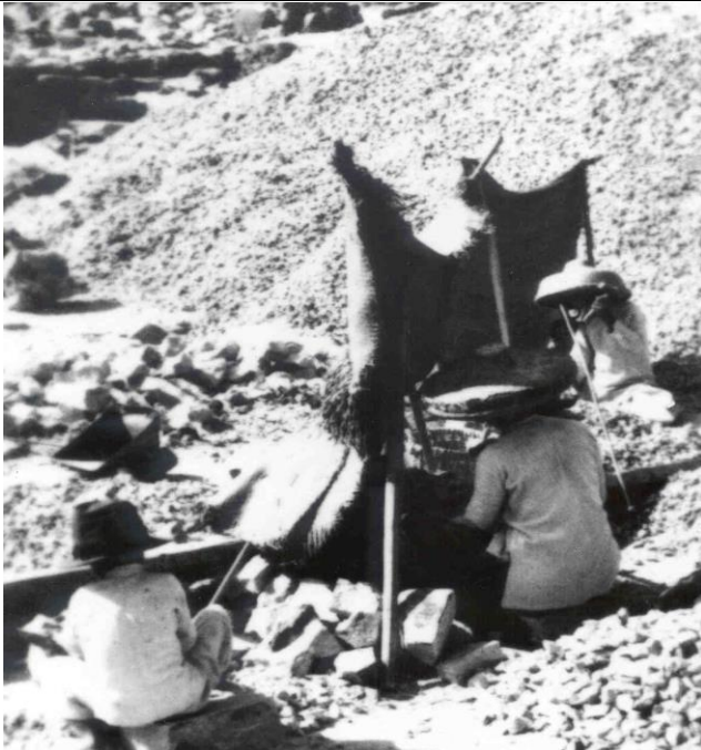
Manual breaking of rock blocks into aggregates 1950s to 1960s
