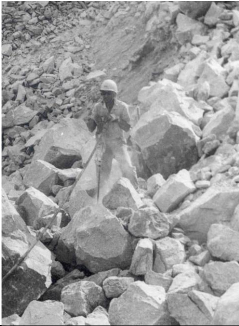
Drilling hole in large block by jackhammer ca 1960s
