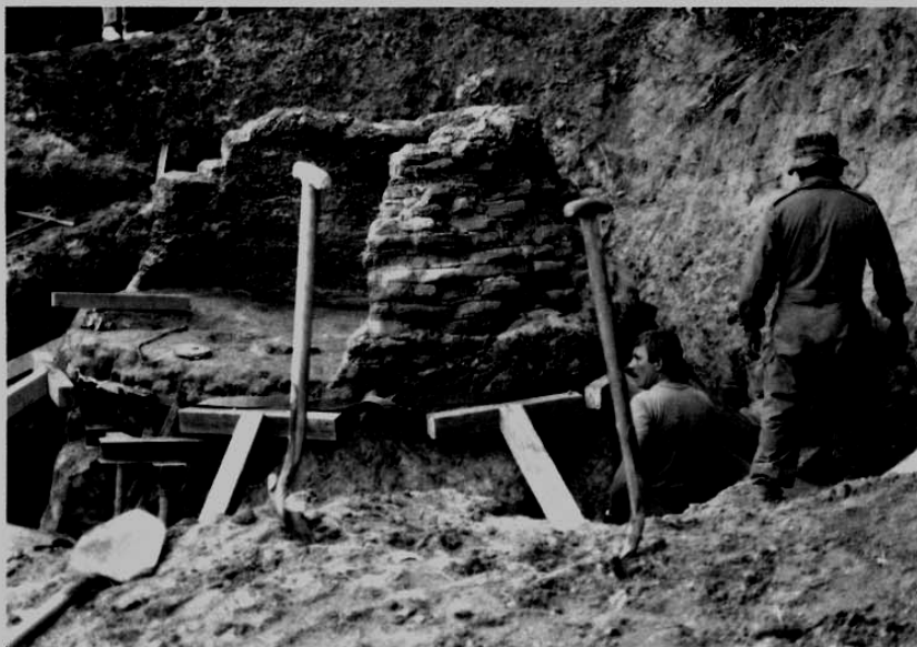
Figure 11.2 -- Trench around the kiln with supports in place.
