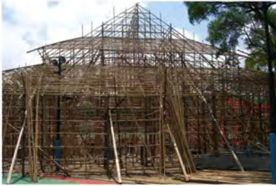
竹棚搭建 Construction of bamboo shed theatre
