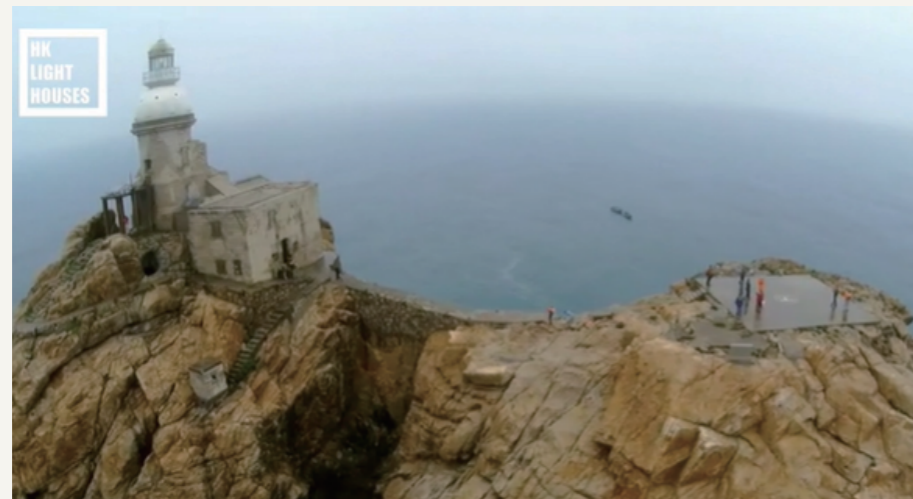
Video footage of Gap Rock Lighthouse
